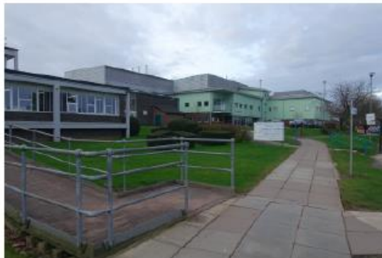
4. Pedestrian Route to Entrance 6
